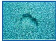
Remove all loose materials from damaged area
