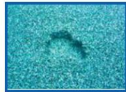
Remove all loose materials from damaged area
