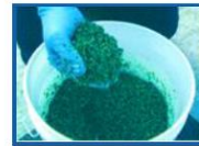
Mix the granules and polyurethane together in the bucket
