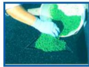
Overfill the hole to allow for compression
